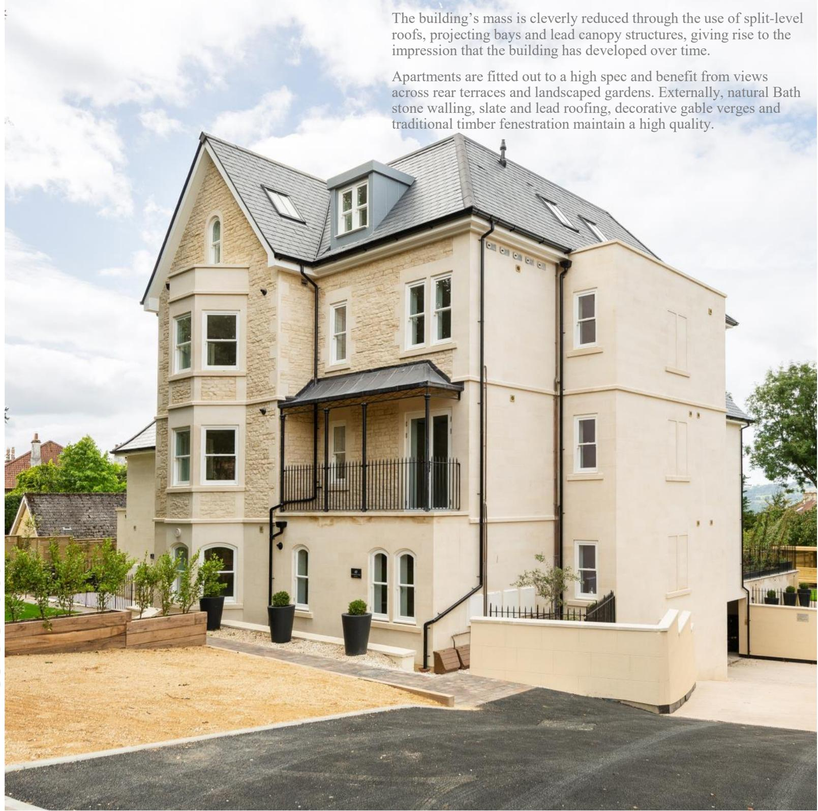
The building's mass is cleverly reduced through the use of split-level roofs, projecting bays and lead canopy structures, giving rise to the impression that the building has developed over time.
